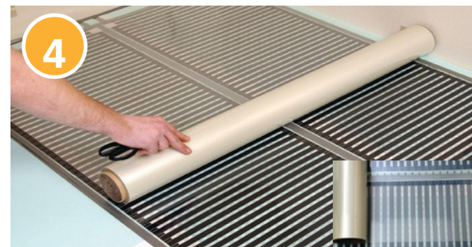
Cover the total ECOFILM PRO installation with POLYESTER VAPOUR BARRIER (available separately).
