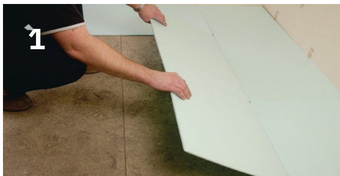
Lay the ECOMAX-LITE Thermal Insulation (available separately) in a "brick work" pattern and fix with adhesive tape.
