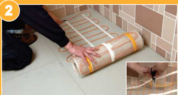
2. Roll the mat onto the floor. When you reach the end of a row, cut the backing mesh and turn the mat through 180° and position the next strip adjacent to the first.
