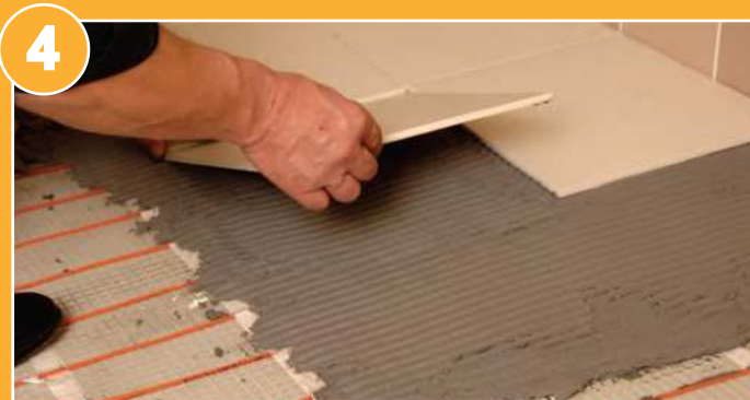
4. Cover with a layer of self-levelling compound/flexible tile adhesive and allow to dry before tiling. Alternatively lay the adhesive and tiles in one step ensuring the cable is totally encapsulated to prevent air gaps.
